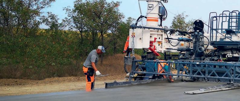
The inset slipform paver is the perfect choice for the cost-effective paving of large concrete surfaces ranging from 4.5 m to 12.0 m wide and 450 mm thick.
