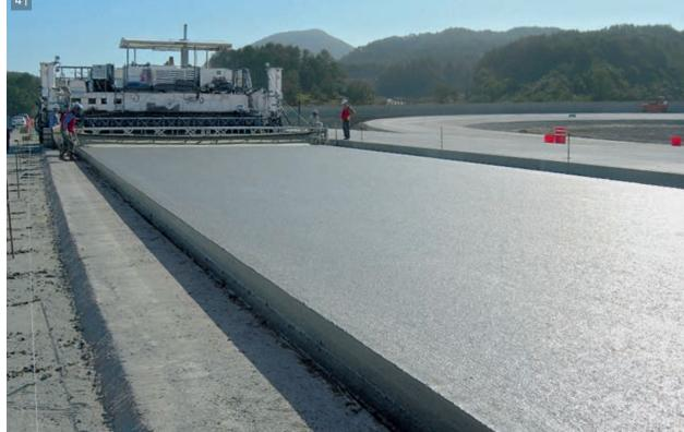
2 The heavy-duty oscillating beam re-moves irregularities in the surface across the full width.
