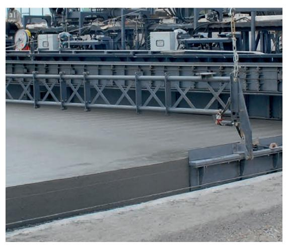
1-2 Economical concrete paving at working widths ranging from 5.0 m to 16.0 m.
