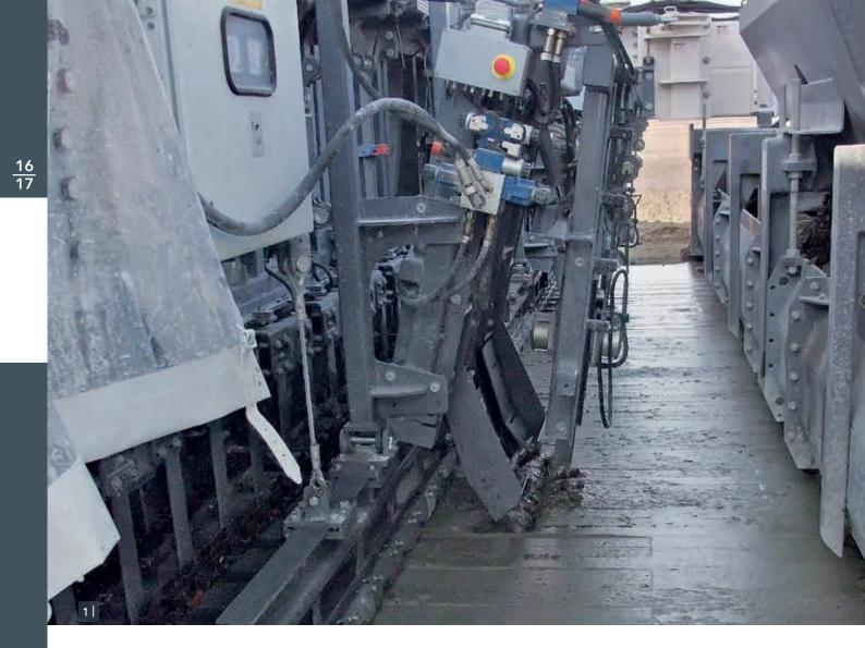
1 The tie bars inserted by the tie bar inserter prevent the slabs from drifting apart.
