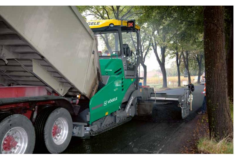
As an alternative to oscillating push-rollers, we also supply PaveDock, our spring-loaded push-bar. This absorbs jolts from the feed vehicle even more effectively and reliably, thus ensuring that they are not transmitted to the finished
